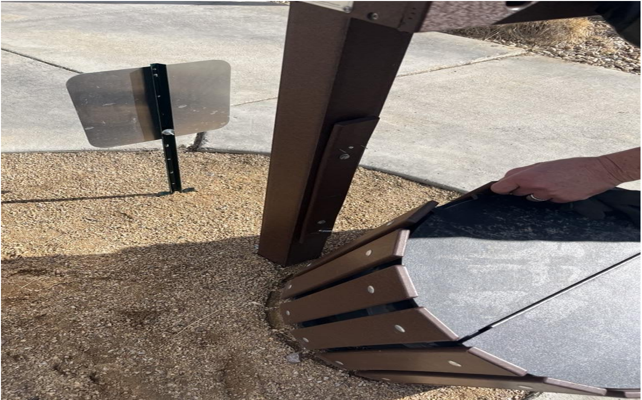
Dog Station at Bason Park was damaged but will be repaired by EDI.
